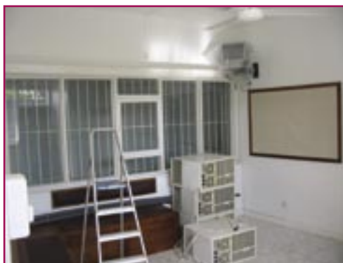
The waiting room takes shape.
